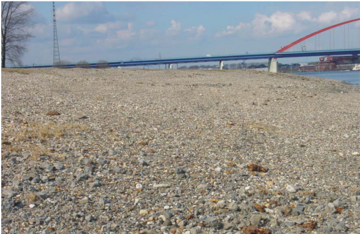
Figure 2: River Rhine at Duisburg after morphological improvement; structures will be created by the next floods and should be maintained
