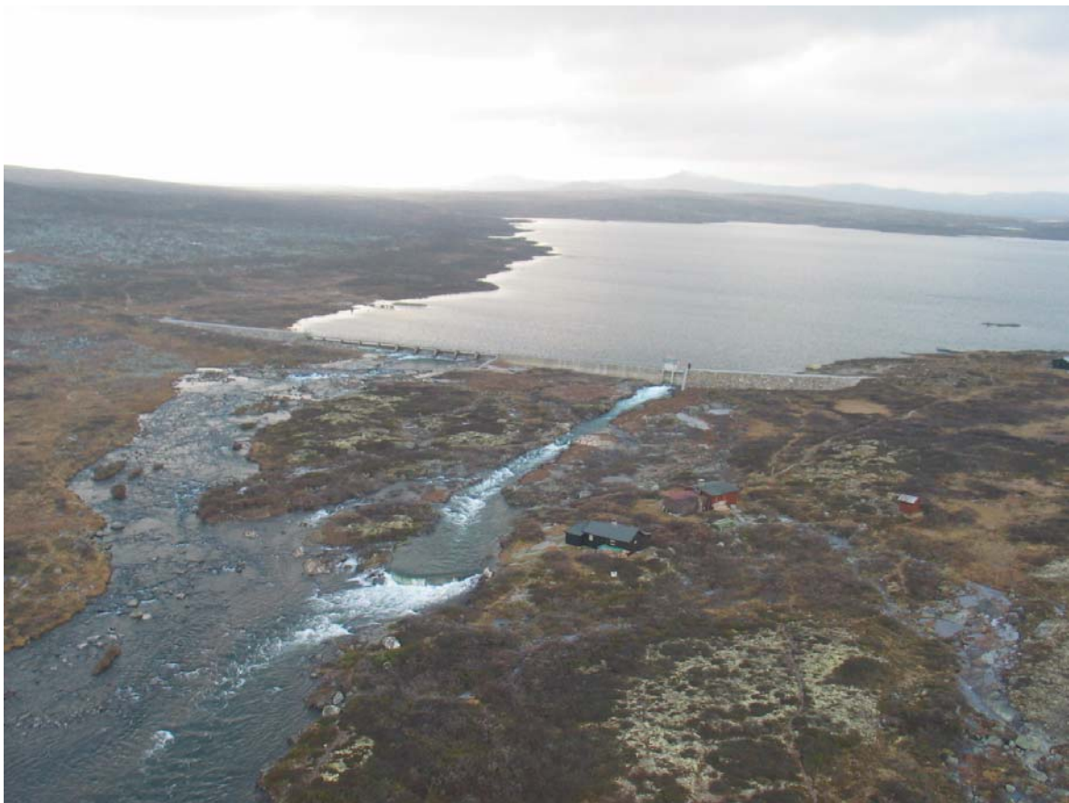
Figure 1: Downstream the dam of the Halneffjord reservoir.
