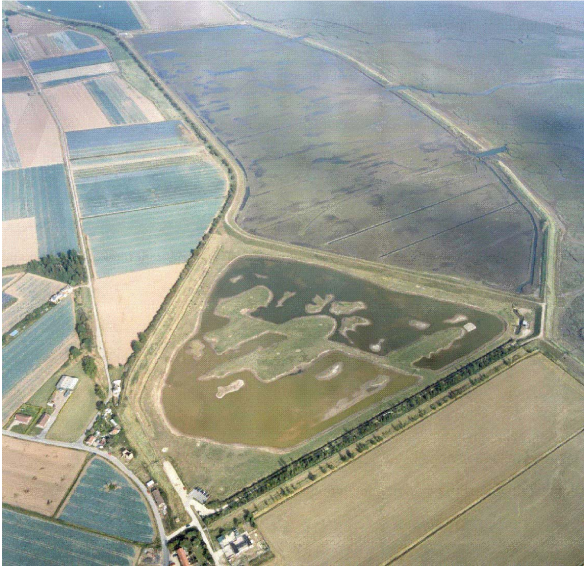
Figure 2: The completed realignment site.
