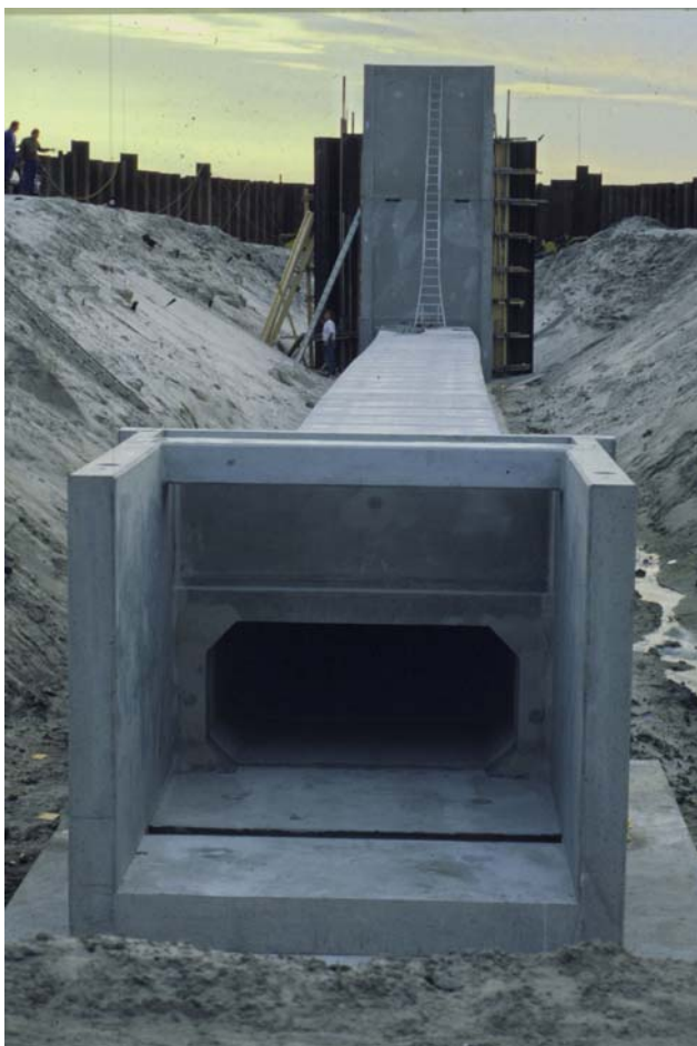
Figure 1: Culvert in the dyke between the Ems-Dollart.
