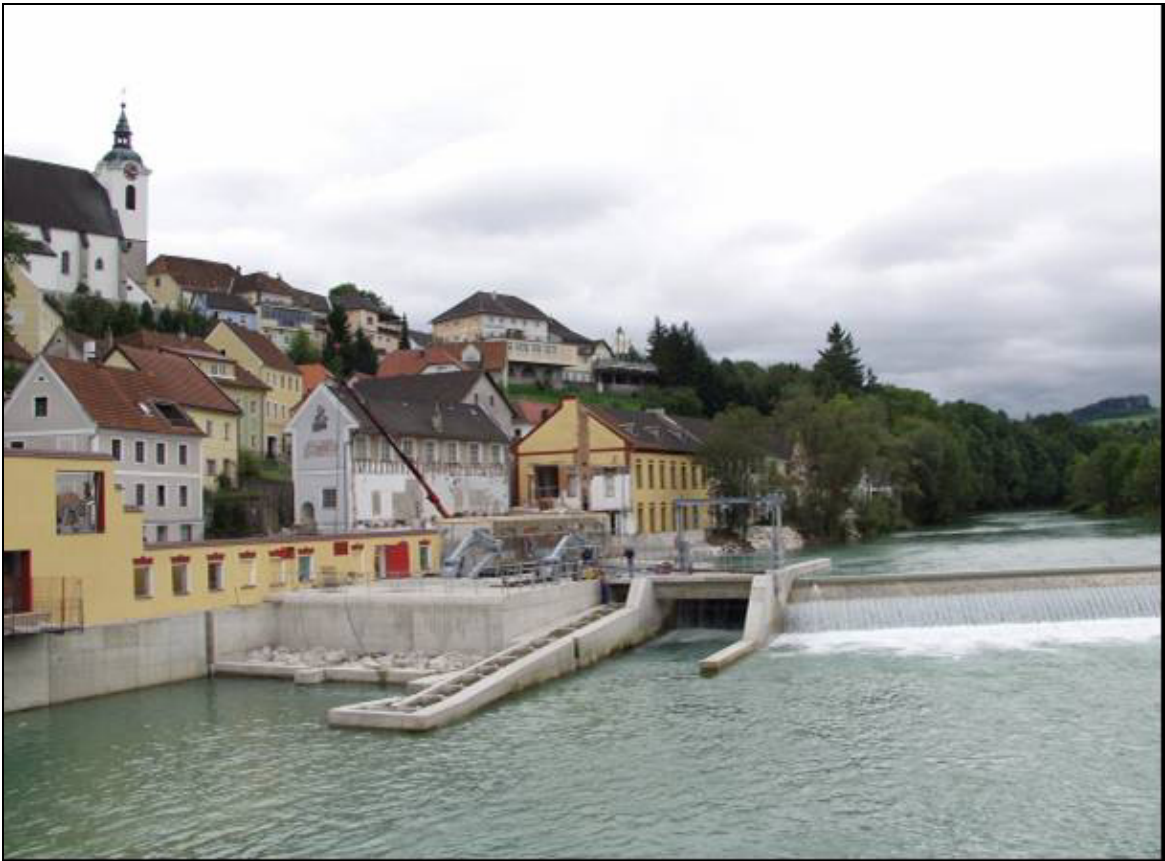
Figure 1: New Steinbach HPP.
