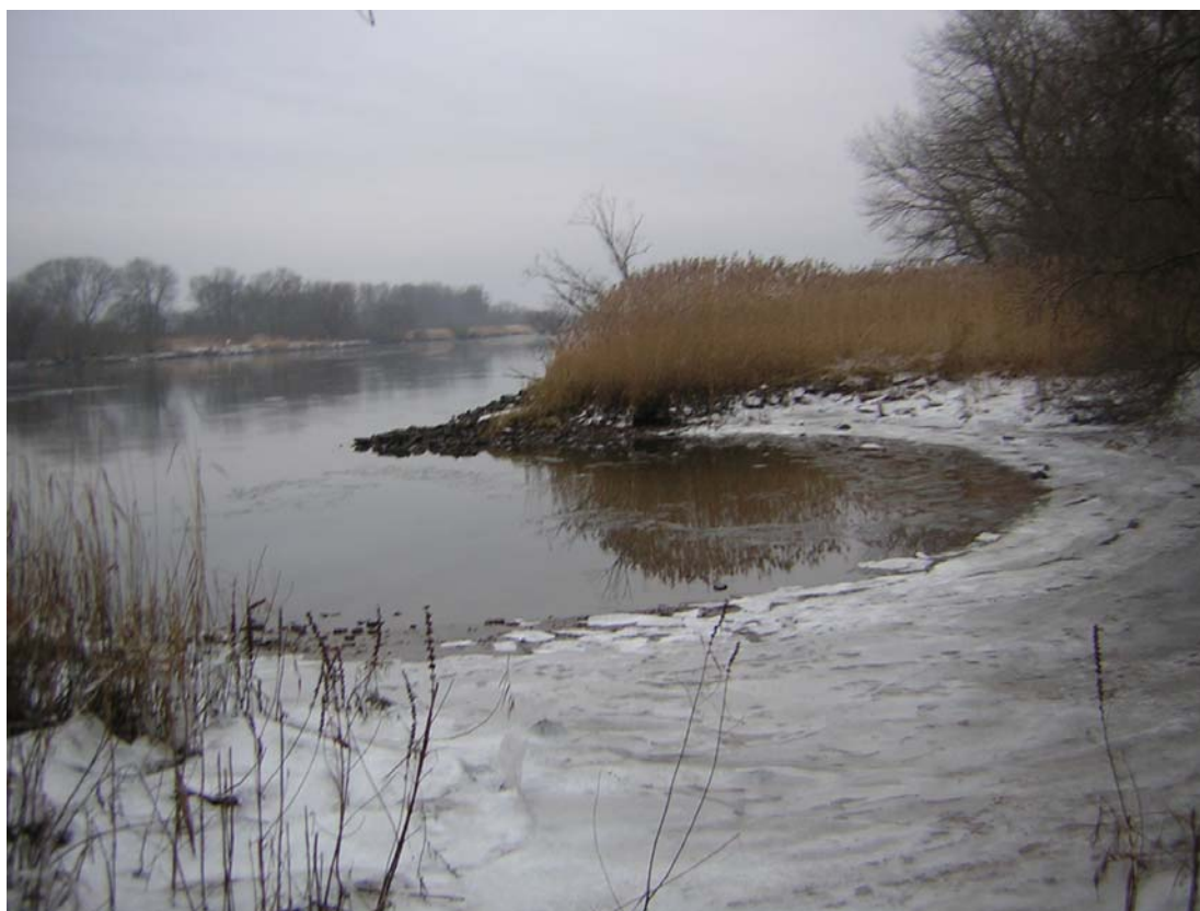
Figure 1: Inlet in the stone filling at the shore of the limnetic tidal river Elbe (January 2006, at low tide). ➤ The iced area marks the small-scale mud and sand flat, which appears at low tide. ➤ The course of the interrupted stone filling is visible in the middle of the picture. Approaching from land, tidal reeds infiltrate the stone filling. ➤ The pictured situation can be found in several sections of the river bank in the natural conservation area “Heukenloch”.
