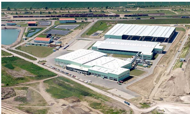
Figure 15 Example of a mechanical-biological treatment plant
