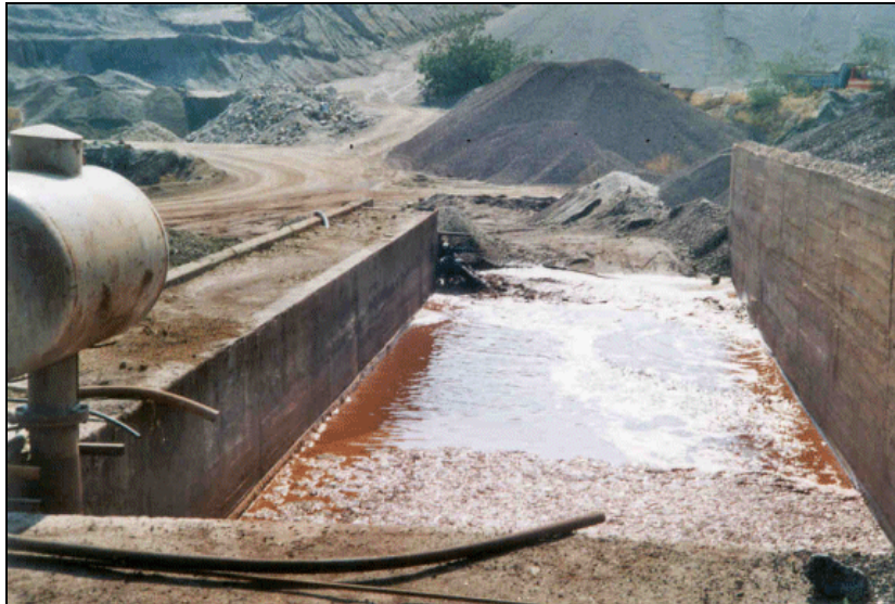
Figure 3.49: Dewatering of tailings in concrete basins [110, IGME, 2002]
