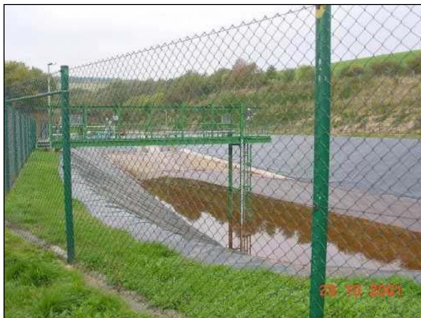
Figure 3.75: Water retention basin of German potash mine
