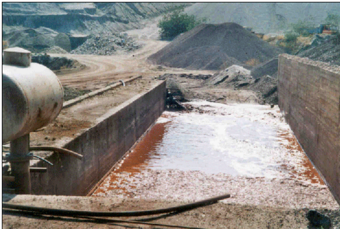
Figure 1.24: Example of a small tailings settling basin
