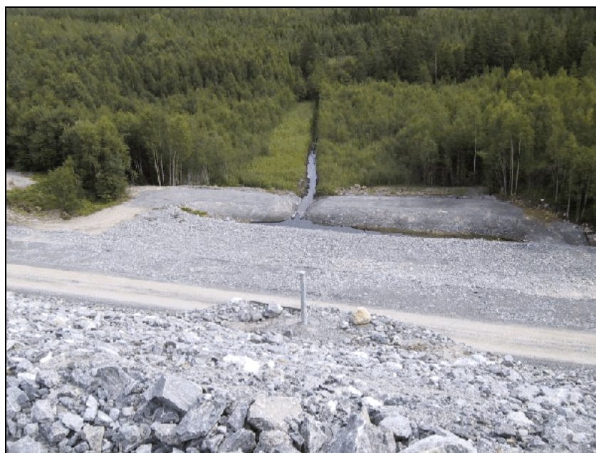
Figure 3.23: Another ditch for collection and flow measuring of seepage water alongside the dam [66, Base metals group, 2002]
