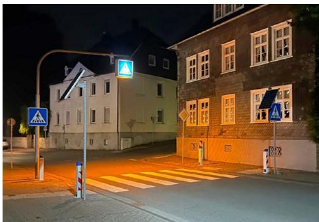
Figure 42: Illuminated pedestrian crossing with laser and LED technology · Source: Blömen VuS
