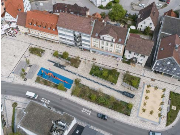
Figure 48: Overview of Obertorplatz, Hechingen Source: Martin Keidel
