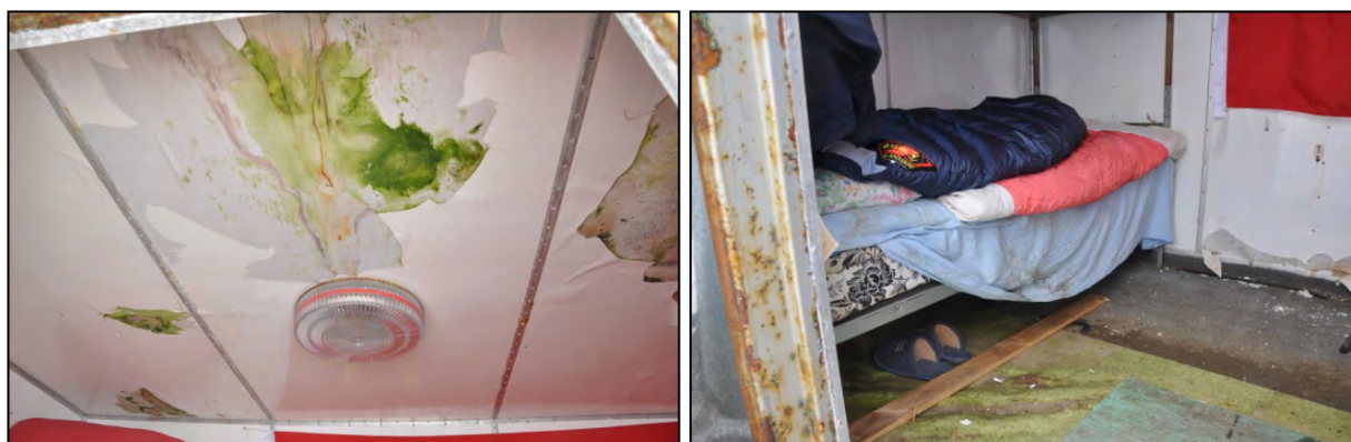
Fig. 36 a & b: Water damage inside the Chinese container (photos: C. Braun, 23.12. 2009 (a) and 16.01.2010 (b)).
