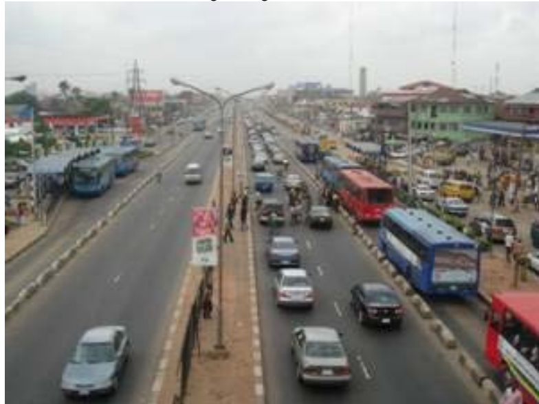
BRT Lite infrastructure in Lagos, Nigeria.
