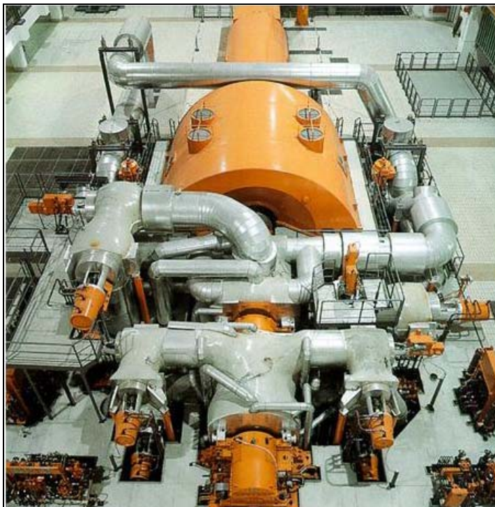
Figure 2.1: Modern steam turbine of a coal-fired power plant [165, NWS, 2001]
