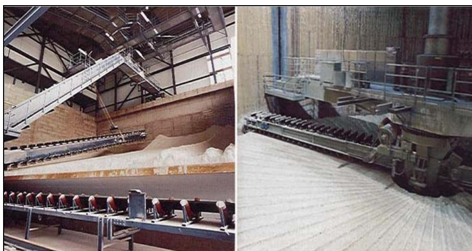
Figure 4.23: Closed gypsum storage facilities [94, Umwelt + Technik, 2000]
