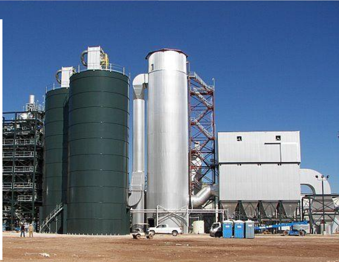
Figure 1 Typical EPI Fluidized Bed Staged Gasifier
