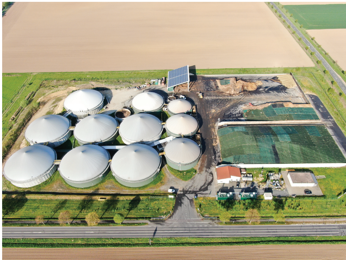
❶ Fig. 3: Rosdorf biogas plant
