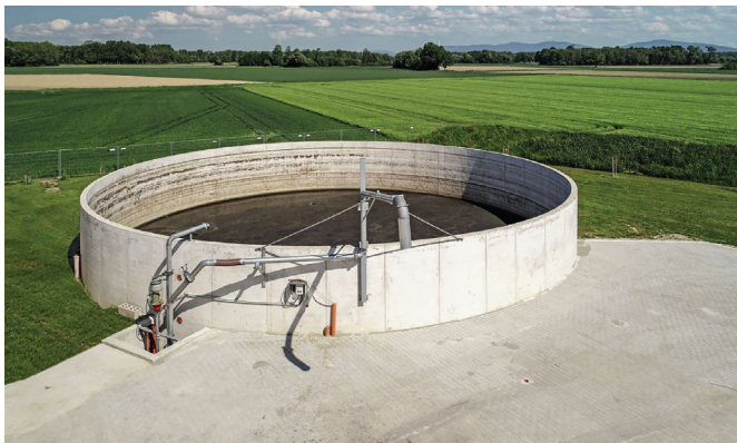
Fig. 5: Ready-mixed concrete containers
