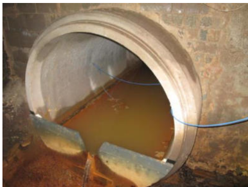
Figure 6: Example of a Triangular Weir
