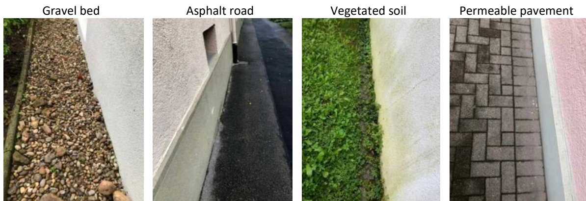
Figure 3: Typical surfaces at the bottom of building façades that accept façade runoff
