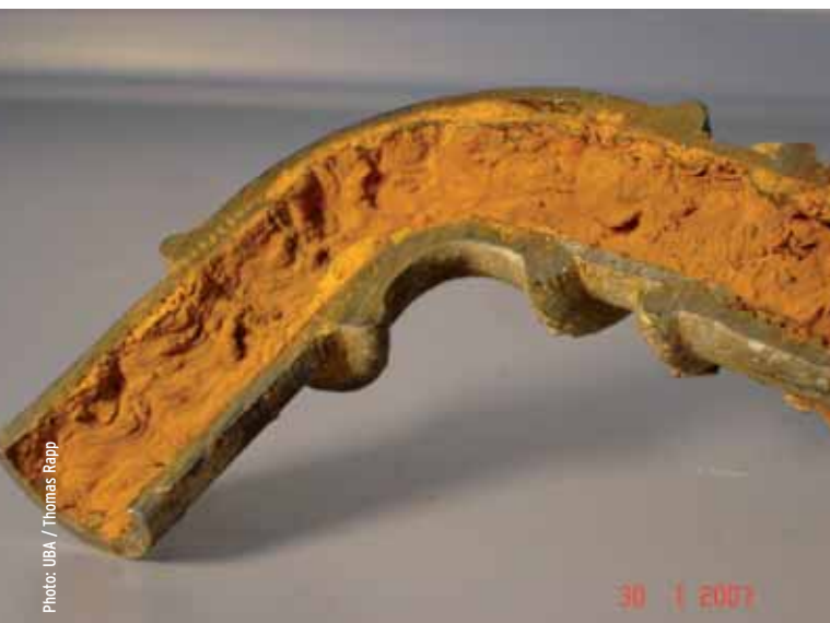
Rusted part on a galvanized steel drinking water installation.
