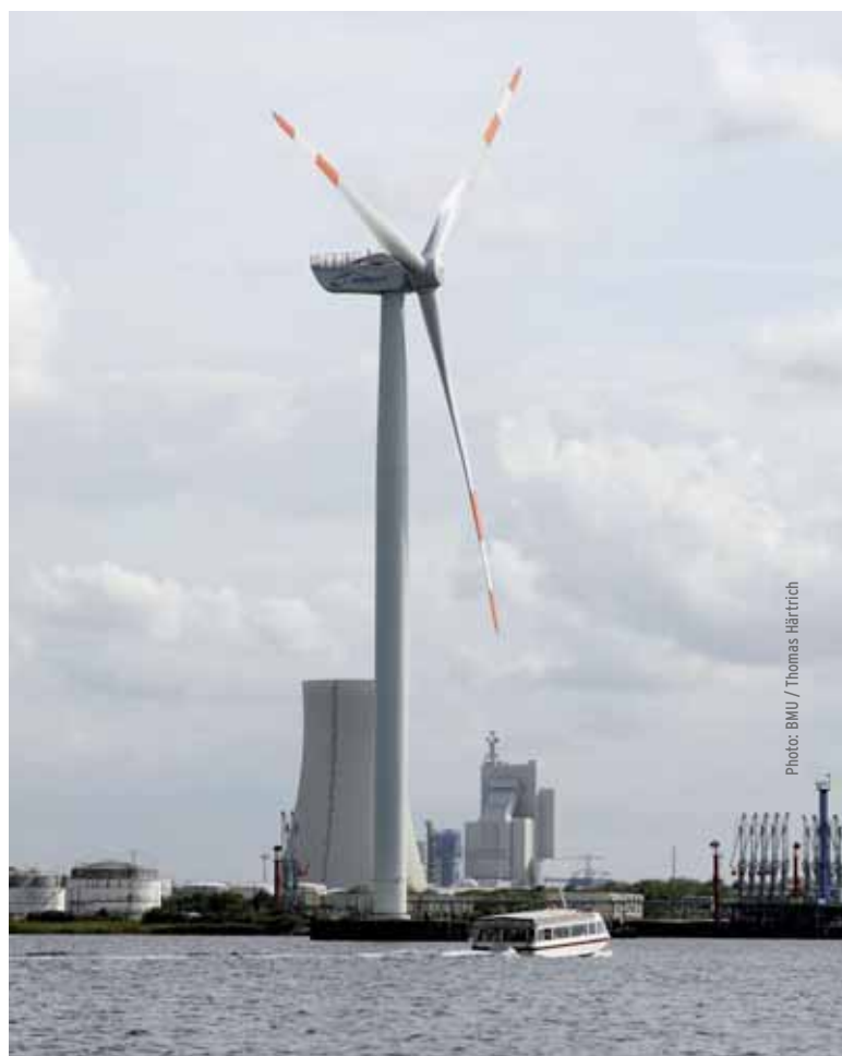
More support needed for wind energy – wind turbine in the port of Rostock.
