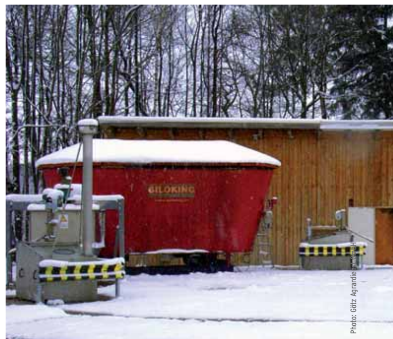
Biogas installation for renewable raw materials...
