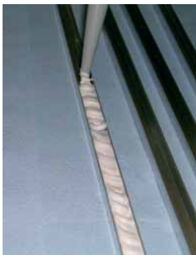
Fig. 5: Applying sealing compound to a standard aluminium channel
