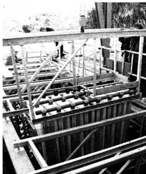
Installation of a membrane filter package at the Markranstädt sewage treatment plant. (Photo: UBA)
