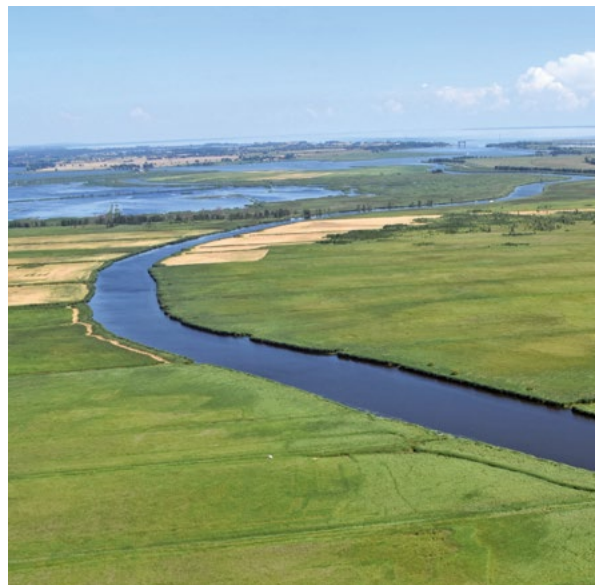
The hydrodynamics prevailing in sections with coastal watercourses are subject to the influence of tides and storm surges. (Photo: © Peter Engelke / stock.adobe.com)
