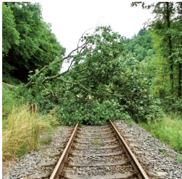
Trees and branches in the track or overhead wires are a potential cause of disruptions to the railway infrastructure. (Photo: © Turner / stock.adobe.com)
