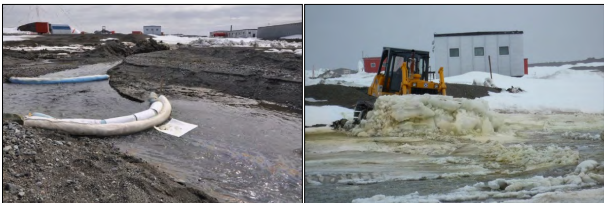
Fig. 59 a & b: (a) Absorbent oil barriers in the mouth of Kiteshbach; on the right the oil film is recognisable behind the oil barriers (photo: C. Braun, 31.12.2009), (b) snow contaminated with diesel fuel is pushed into the sea on 21.12.2009 (photo: A. Nordt).
