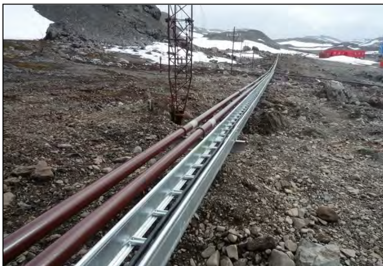
Fig. 30: New fuel pipelines connecting the fuel storage tanks with the station (photo: A. Nordt, 27.02.2010).
