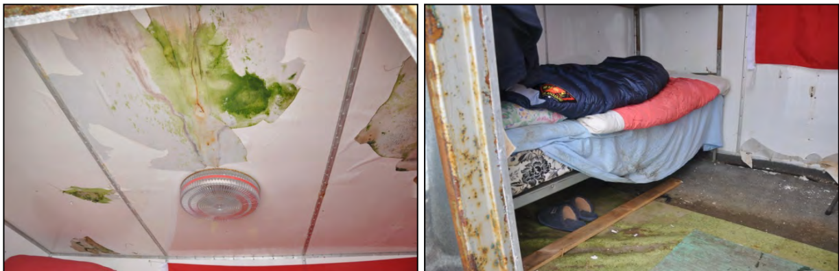
Fig. 36 a & b: Water damage inside the Chinese container (photos: C. Braun, 23.12. 2009 (a) and 16.01.2010 (b)).
