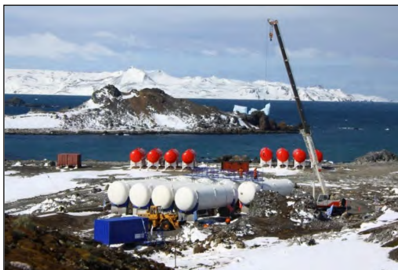
Fig. 29: New fuel tanks belonging to Great Wall Station, set up in the 2009/10 season (white, in foreground) and old tanks to be replaced (red, in background; photo: A. Nordt, 06.02.2010).
