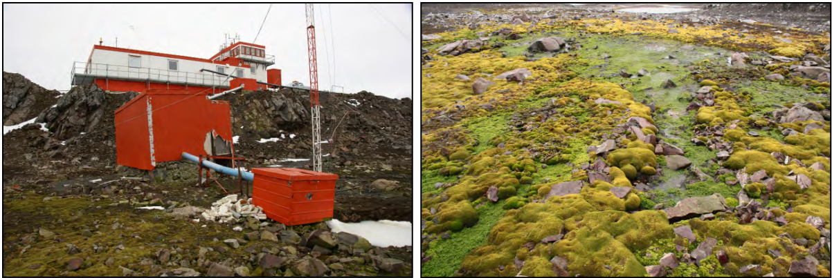
Fig. 56 a & b: Situation at the wastewater treatment facility behind the airport tower: (a) damaged sewage container (photo: A. Nordt, January 2011); (b) noticeably vigorous growth of algae (e.g. Prasiola crispa ) and moss in the immediate vicinity of the sewage system (photo: S. Janowski, January 2011).
