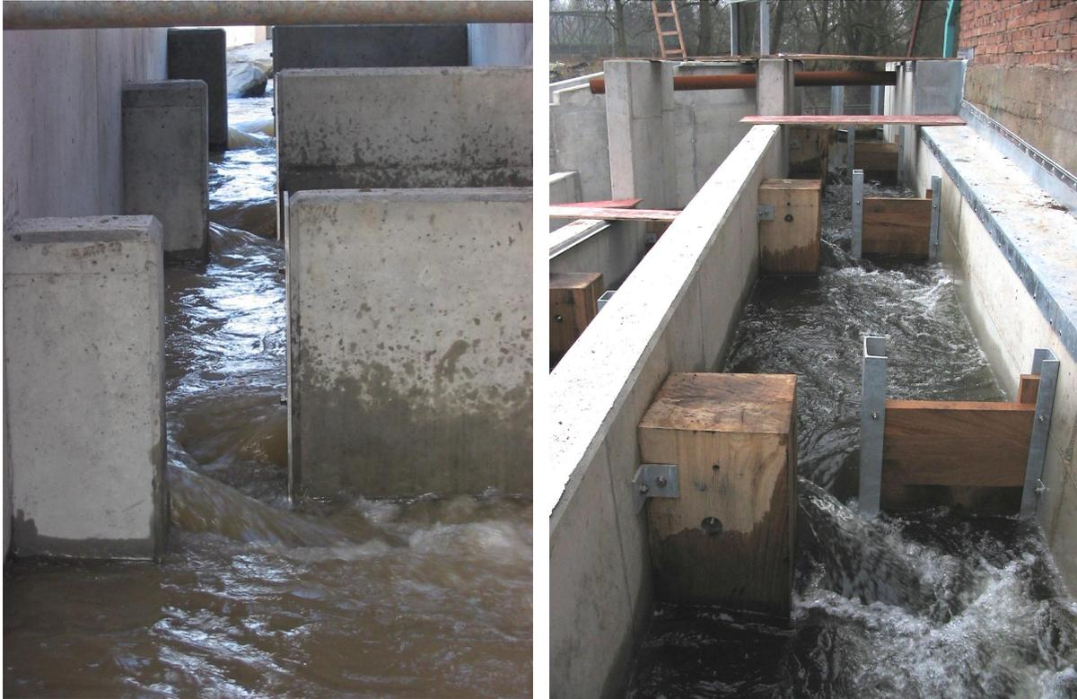
Abb. A.28: Links: Vertical-Slot-Pass Klinkelsche Mühle in Gießen (Hessen).
