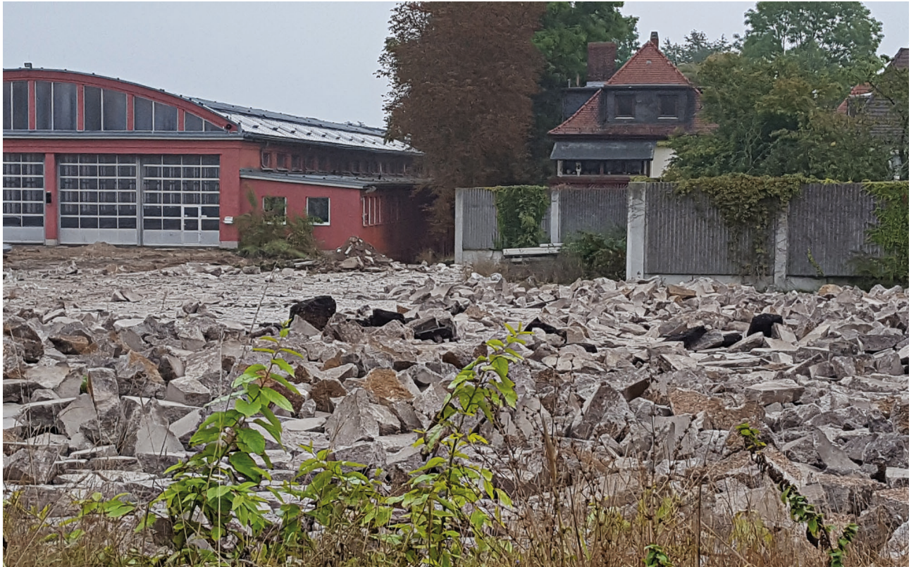
Demolition of a concrete traffic area
