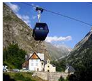
Figure 9: Example of a cable car, connecting the mountain areas with the lower part of the valley.
