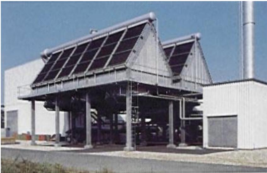
**Figure 2.15: Example of an air-cooled condenser for condensation of turbine exhaust steam [tm111, BDAG, 1996]**
