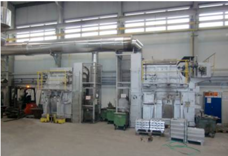
Fig. 14: The exhaust systems of the four furnaces on JURA CAST are connected with heat exchangers. These transmit the heat of the hot gases from the melting process to the heating circuit (source: IfG)
