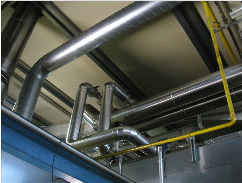
Fig. 6: Thermal oil pipes for water-based paint drying (source: IfG)
