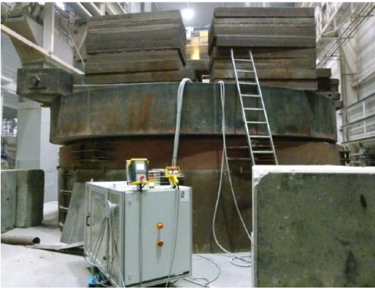
Fig. 18: Control of the oxy-fuel diffusion burner (source: IfG)
