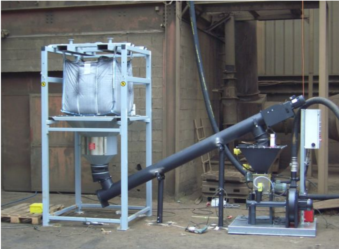
Fig. 10: View of an installation (source: IfG)
