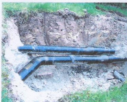
Preparation of Pipelines for wall thickness gauging
