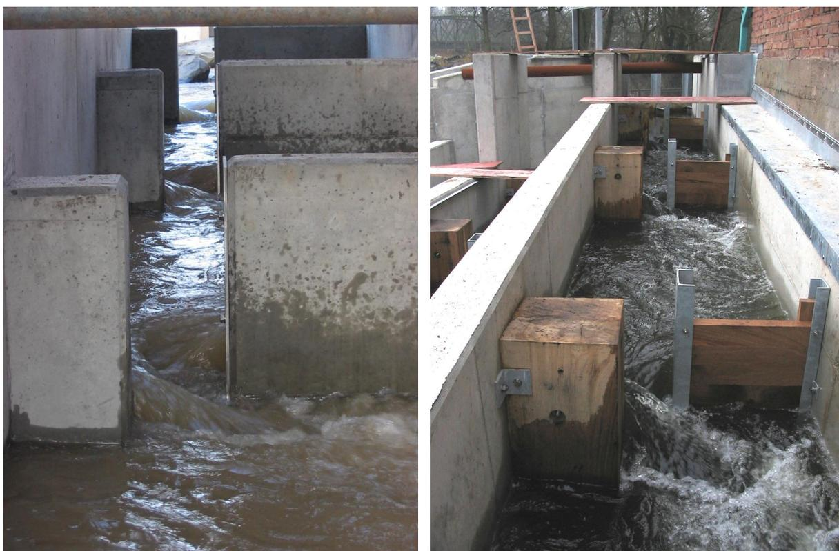
Abb. B.28: Links: Vertical-Slot-Pass Klinkelsche Mühle in Gießen (Hessen).
