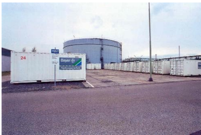
Figure 2: Storage of parts for mobile protection
