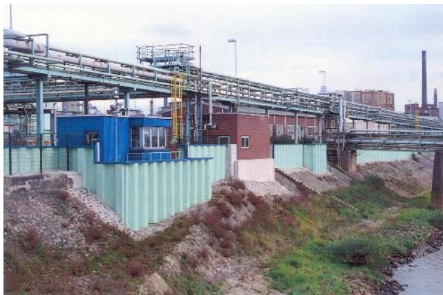
Figure 1: Flood protection wall
