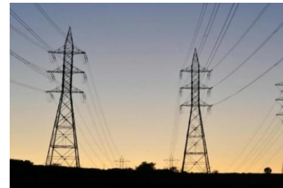
Access to electricity
