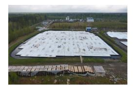
Open lagoon at Krasnyi Bor landfill after covering with an anti-filtration coating in 2017
