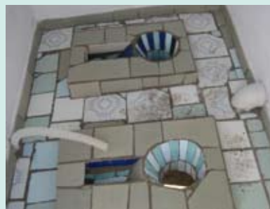
Self-made squatting slabs of a double vault UDDT.
