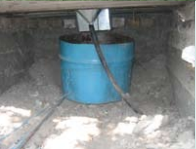
Single vault UDDT: faeces are collected in the blue bucket, which can be moved out on rails.
