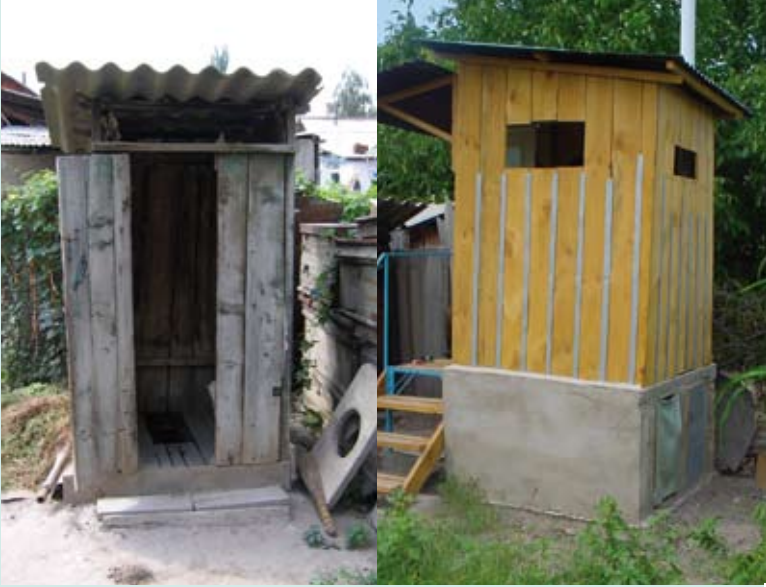
Old and new: pit-latine (left) and UDDT. Faeces chamber doors are on the right side.
