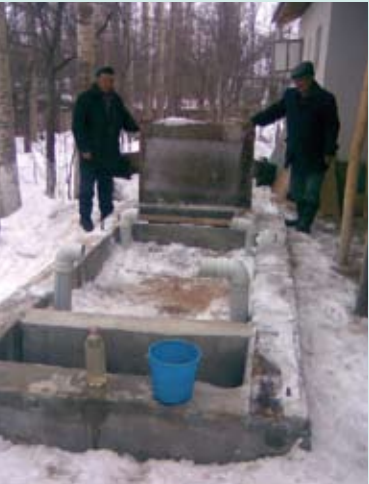
Constructed wetland in Jetygen. The filter never froze even at outside temperatures of -20°C.
