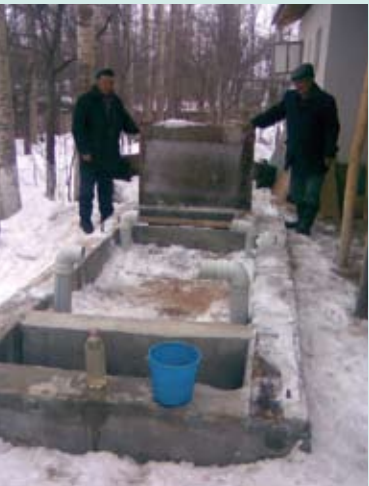
Constructed wetland in Jetygen. The filter never froze even at outside temperatures of -20°C.
