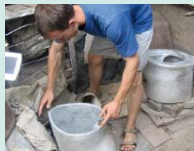
Urine diverting seat riser made from concrete.
