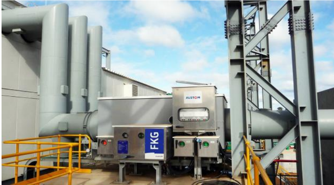
Figure 13: Gas-insulated generator circuit-breaker (Alstom)
