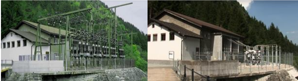
Figure 14: High-voltage transformer station for a hydroelectric power plant
