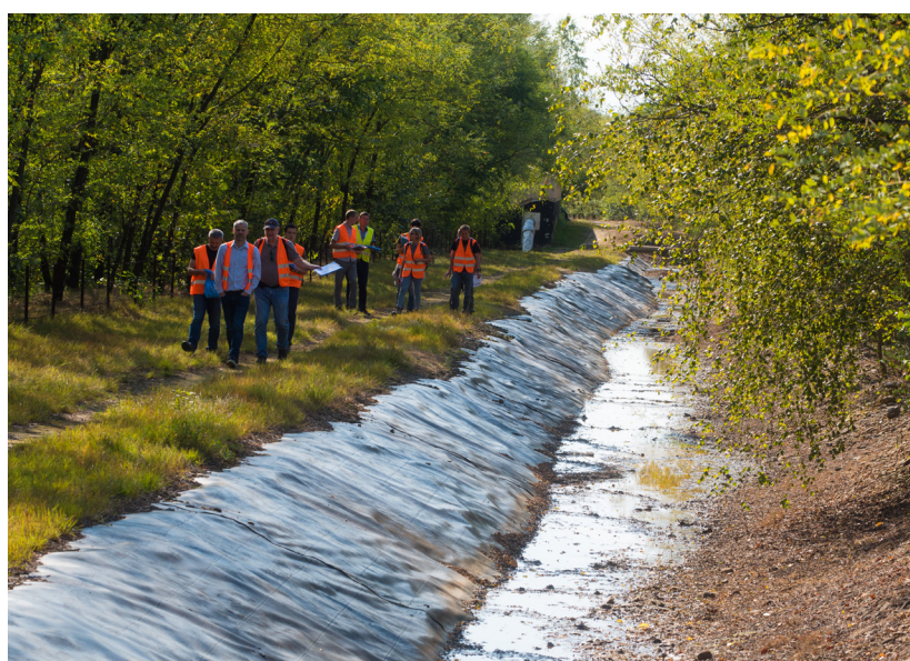
Visual check of the Aurul TMF: main drainage channel with impervious HDP screen (geo-membrane)
