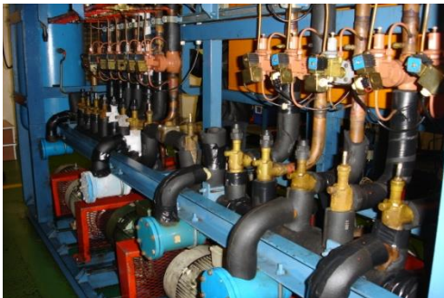
Supermarket refrigeration system
