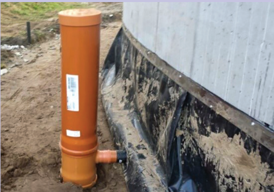
Fig. 9: Drainage pipe with inspection tunnel
