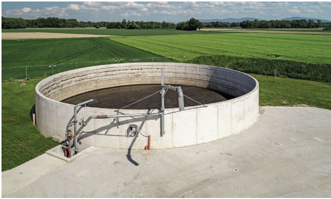
Fig. 5: Ready-mixed concrete containers
