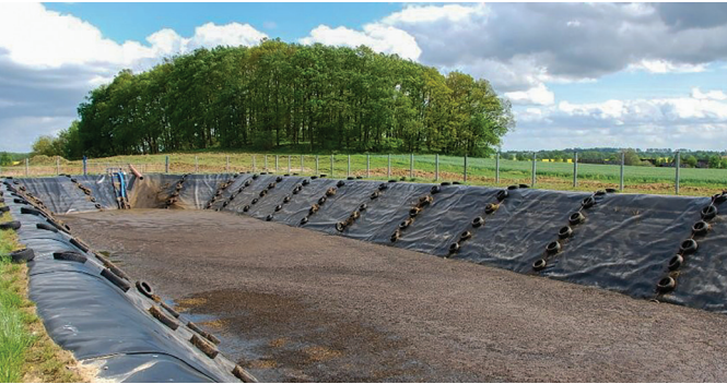
❷ Fig. 4: Ground basin
