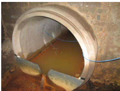
Figure 6: Example of a Triangular Weir
