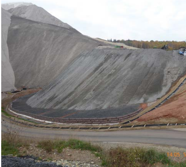
Soil covering of a salt waste dump
