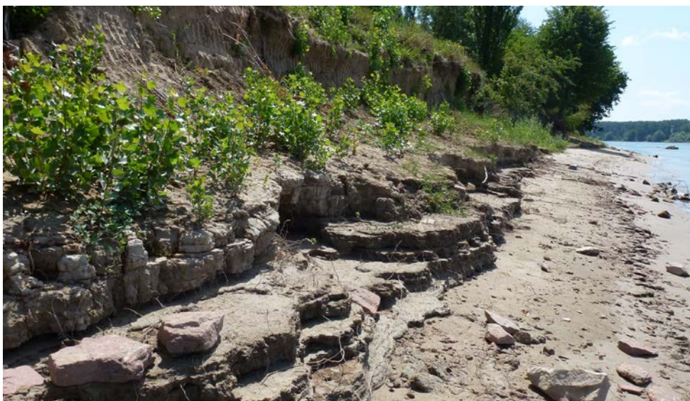
A bank section from which all rocks that had formerly served protection purposes and were no longer needed were removed. An ecologically valuable terrace has formed.
