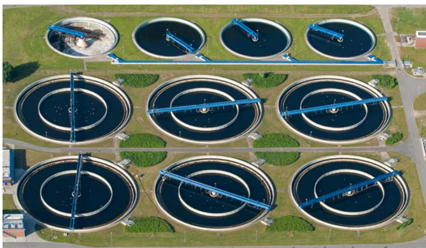
Sedimentation tanks of the Hetlingen wastewater treatment plant in Schleswig-Holstein
