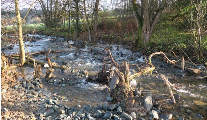
Reshaping the straightened riverbed (having a deepened and narrow profile and almost completely lacking buffer strips) into a structurally rich multi-bed channel, with small islands forming, watercourse widening and banks flattening, with deadwood and rocks for inherently dynamic development
