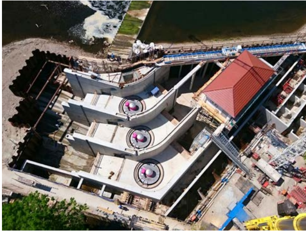
Aerial view of the Öblitz hydropower plant when under construction (one can see three turbine channels and the fish ladder to the right)
