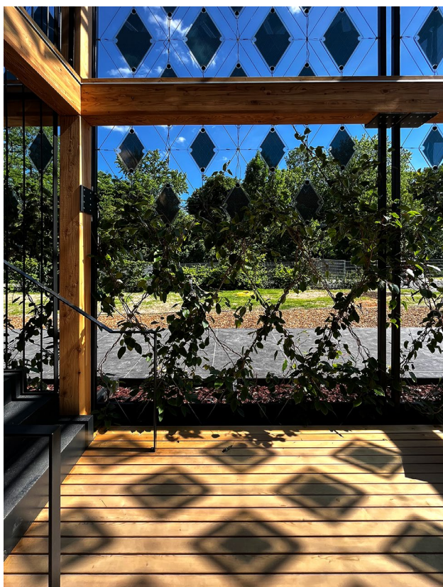
Combination of PV elements and a façade made of reused wood
