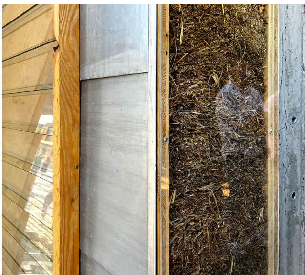
Wall structure using straw insulation
