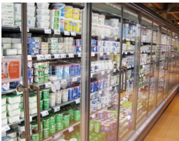
Display cabinet of a transcritical CO 2 refrigeration plant in a supermarket.
