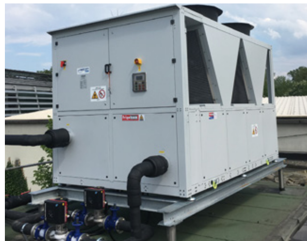
A chiller which uses R-290 (propane) to refrigerate Munich's wholesale market.
