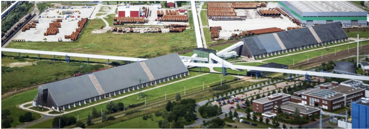
Figure 7 Storage halls for fertiliser with conveyor belt connection to terminal in the port of Rostock
