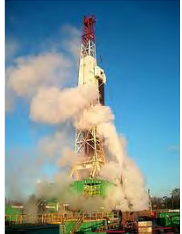
The deep well drilling tower in Unterhaching, Germany
