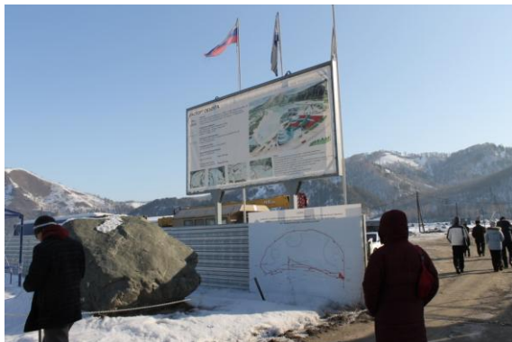
Construction site in the Altai mountains
