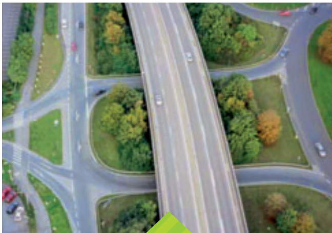
FIG. 2 THE RAPID INCREASE IN ROAD TRAFFIC AND THE DENSITY OF REGIONAL TRANSPORT NETWORKS GO HAND IN HAND
