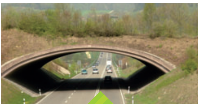
FIG. 3 A GROWING NUMBER OF GREEN BRIDGES PROVIDE WILDLIFE CROSSINGS
