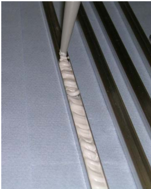
Figure 3-1: Applying sealing compound to an aluminium standard channel
