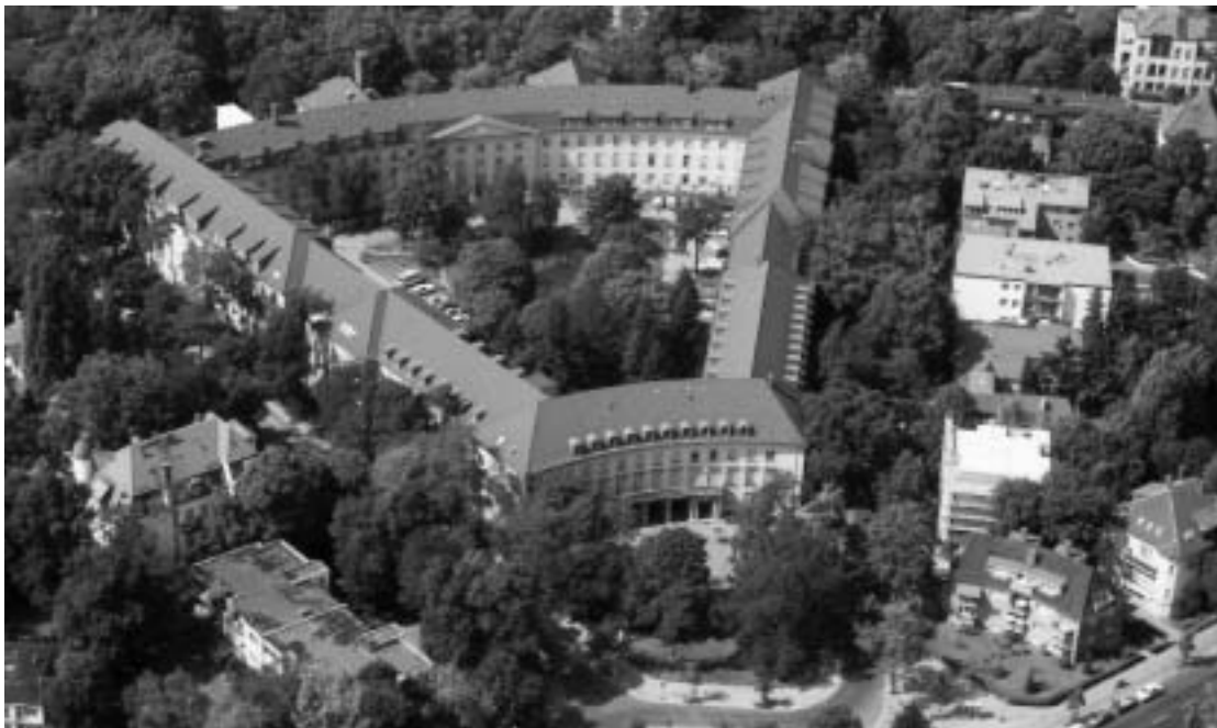
The headquarter of the Federal Environmental Agency in Berlin, Bismarckplatz 1. (Photo: UBA)
