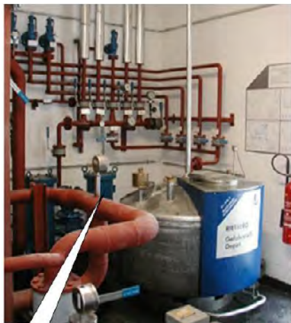
Figure 4.27: Pumping station number 2 with a filter and a waste container for cleaning the filter [50, Germany, 2006], [51, EuLA, 2006]
