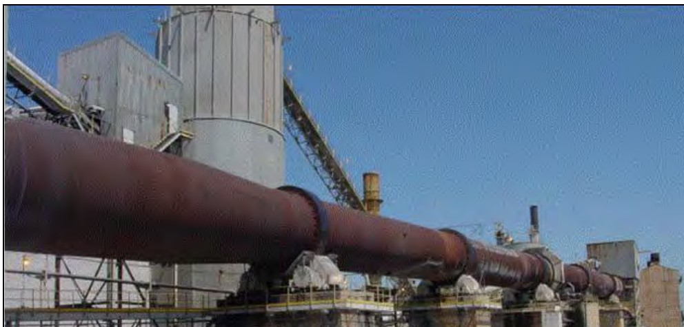
Figure 2.31: Example of a long rotary kiln used in lime manufacture [44, EuLA, 2006]
