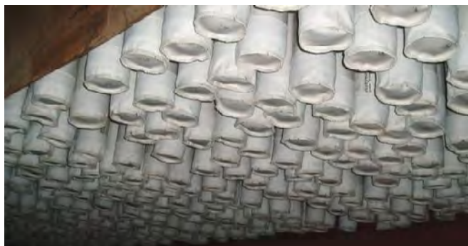
Figure 1.60: Example of a fabric filter and filter material used in a cement plant in the UK [82, CEMEX Rugby UK, 2006]
