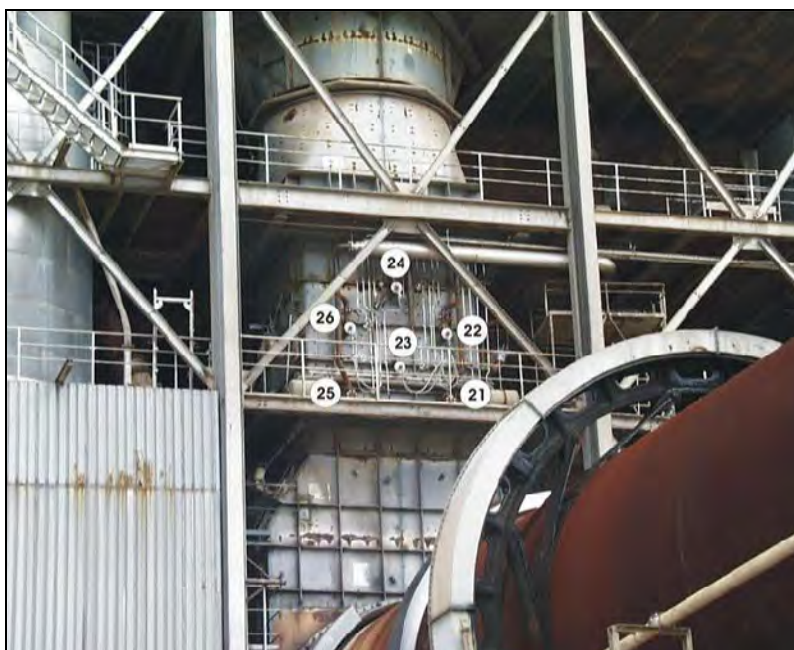
Figure 4.8: High efficiency SNCR and place for injection of ammonia water via lances at places Nr. 21 to 26 [76, Germany, 2006]
