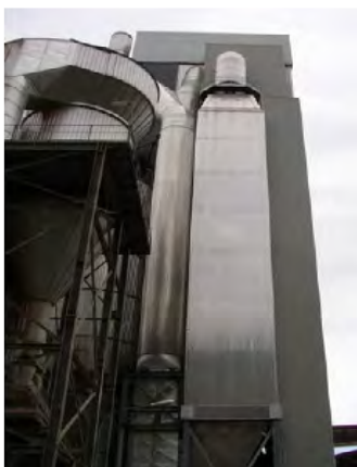
Figure 1.66: Example of an SCR installation [140, Italy, 2007]
