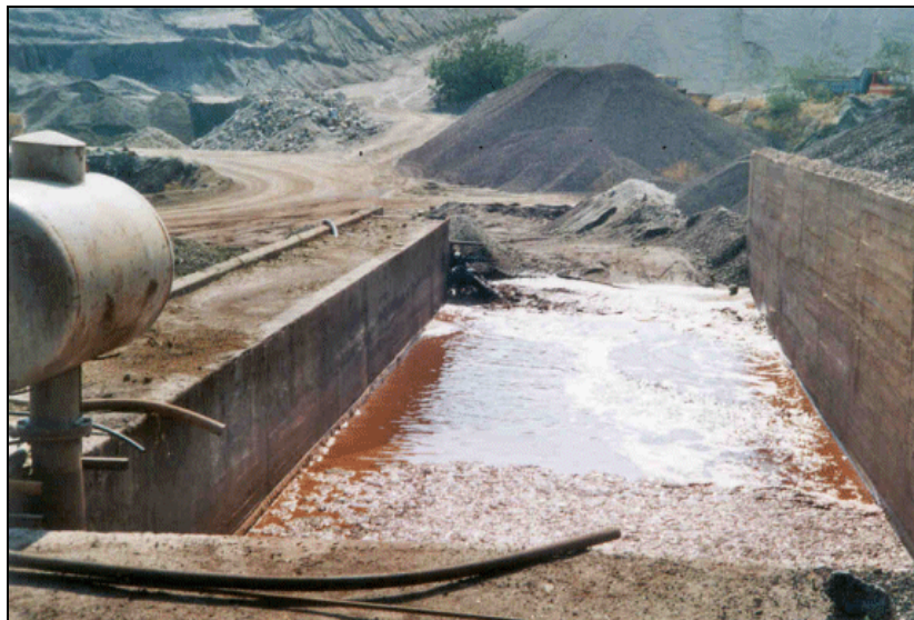
Figure 3.49: Dewatering of tailings in concrete basins [110, IGME, 2002]
