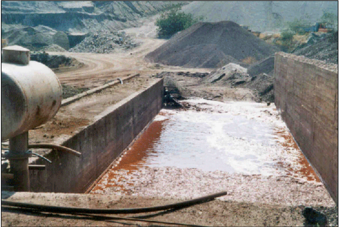
Figure 1.24: Example of a small tailings settling basin
