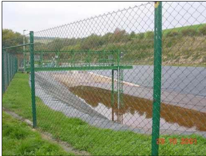
Figure 3.75: Water retention basin of German potash mine
