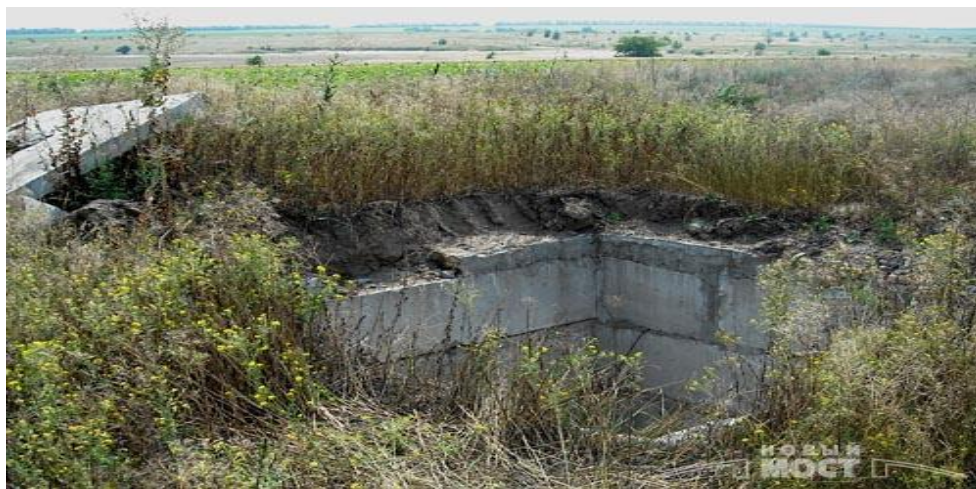
Figure A 1.3: Abandoned tailings in Dnipropetrovsk, Ukraine
