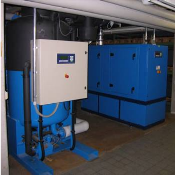
Figure 62: Combined heat, power, and cooling system (left-hand side picture, right-hand side machine) and absorption type refrigeration system (left-hand side picture, left-hand side machine) for air conditioning of a commercial building (right-hand side picture) (Weidner 2008)
