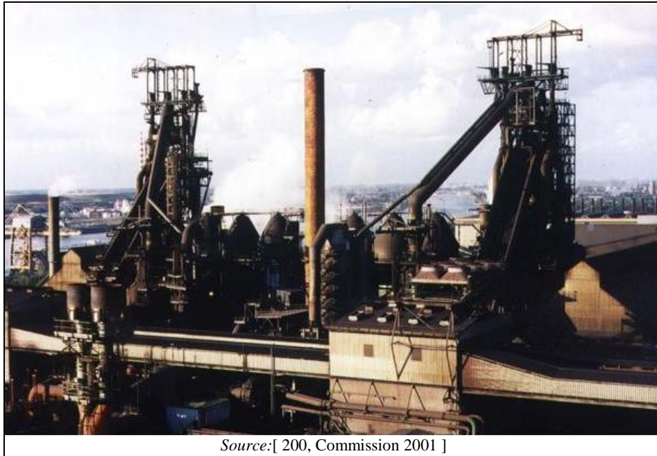
Figure 6.1: General view of two blast furnaces with three hot stoves each and the stack for the waste gas from the hot stoves
