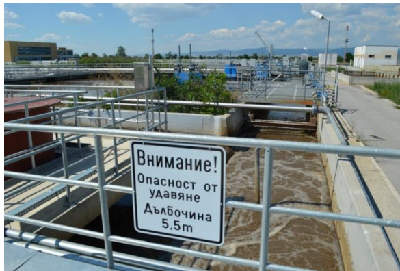
Wastewater treatment in Sofia. Photo: INTECUS GmbH
